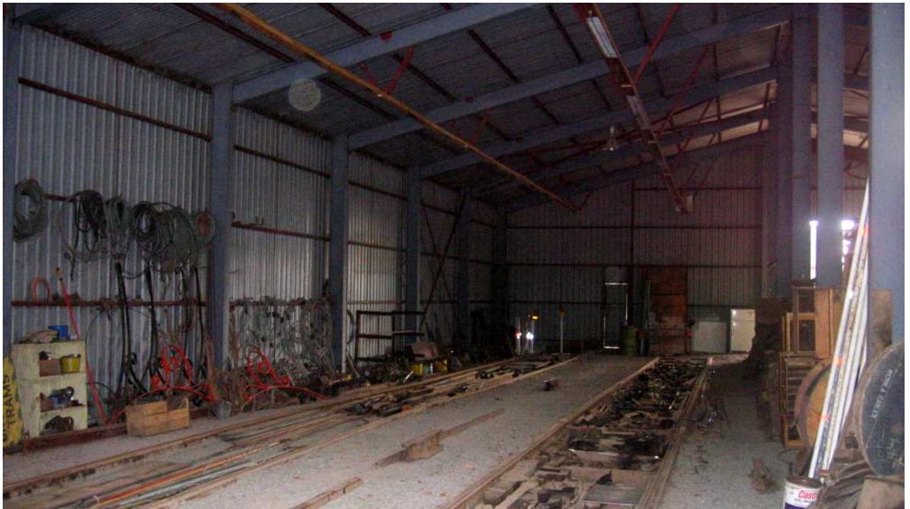
Six and seven roads empty of trams. An unusual sight. The accumulations of thirty years are being worked through. Shelving will be installed along the side wall. The new overhead is also evident on seven road. 2/9/2006
