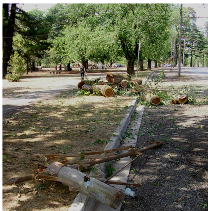
The remains of the broken pole following the storm on New Year's evening.
