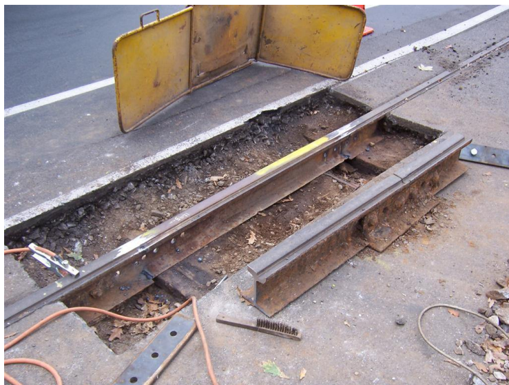
Left: A replacement section of rail has been welded into place and awaits the fishplates.
