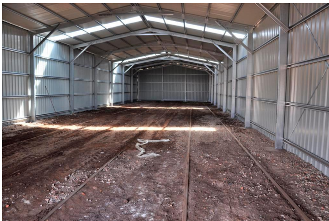
Above: The new shed awaits tramcars. Photo: Alastair Reither 17/2/12
