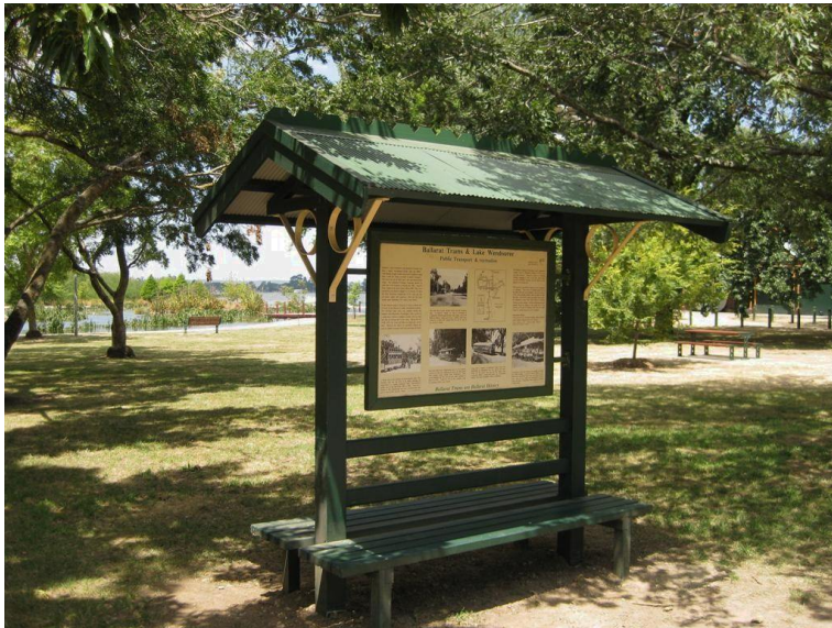
The refurbished shelter Photo: Peter Winspur 27/1/12
