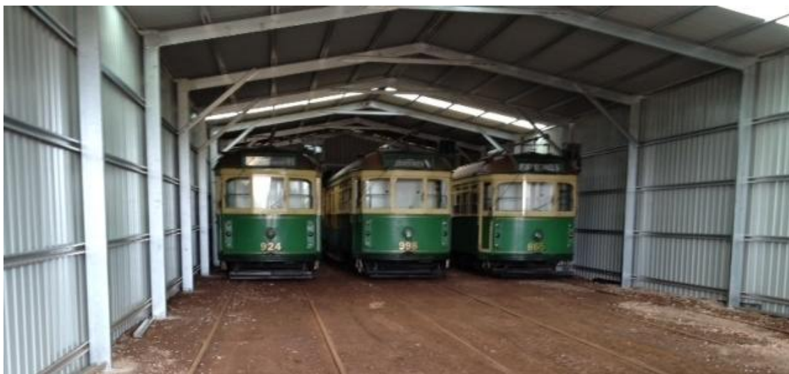
The first trams in our new shed. They had just come in from the rain Photo: Paul Mong 28/2/12
