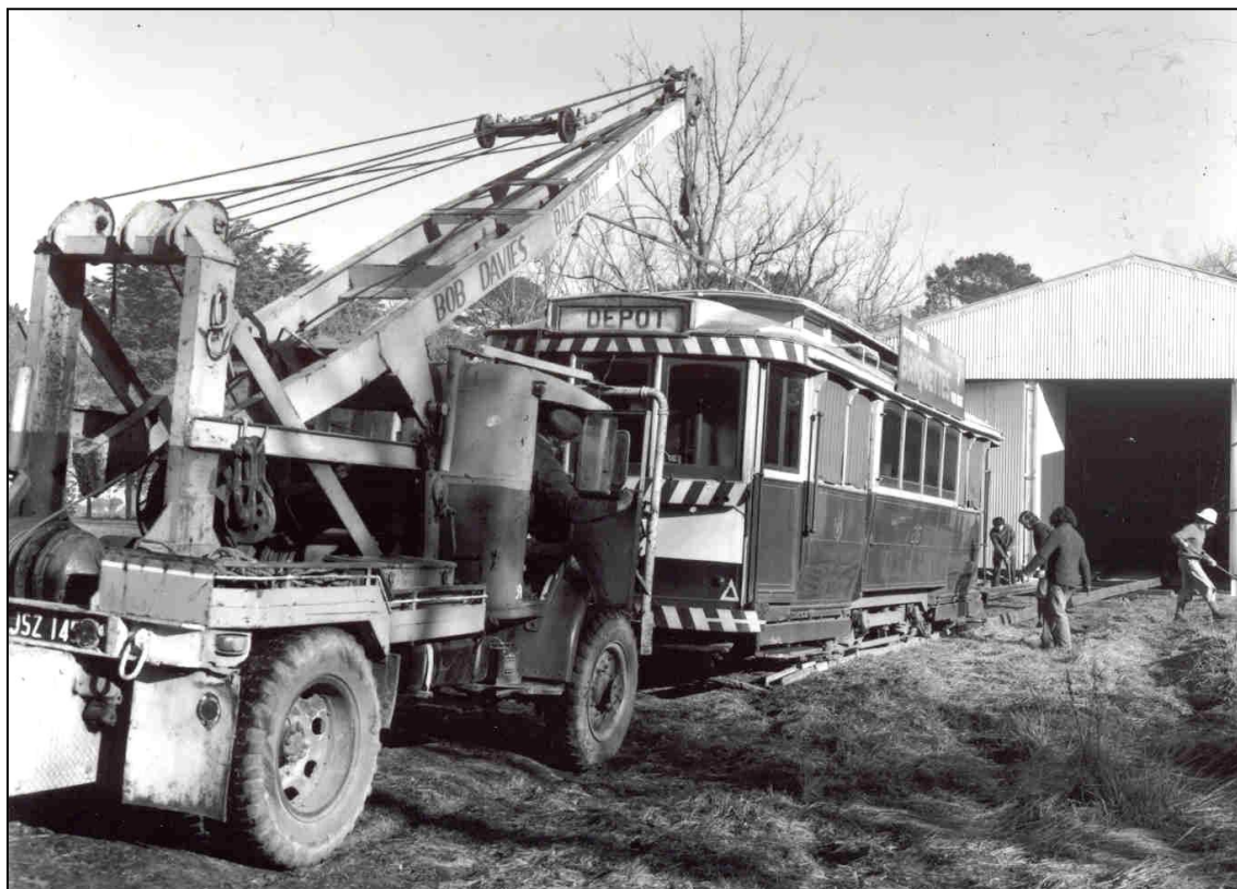
Moving the first tram into the Depot 17 June 1972. Note use of steel channels and rails on their side. Published in The Courier on 19 June 1972.
