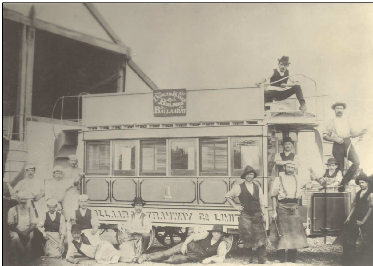
Newly assembled Tram No 1 at the Wendouree Depot This photo was very important during the reconstruction of the tram by the Museum. BTM Collection
