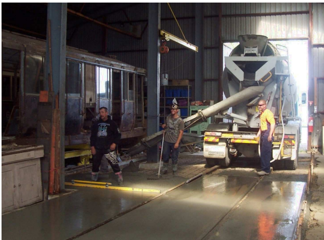
Above: Concreting 5 Road 15/11/2012
