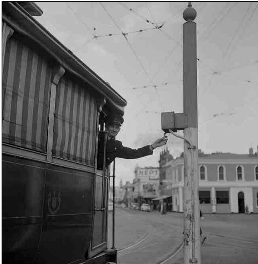
The motorman operates the selector switch at the corner of Sturt and Grenville Streets
