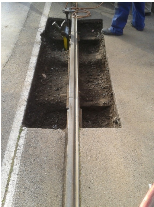
Above: The section of rail needing repair. Some years ago the Museum had inserted a section to repair the original join.
