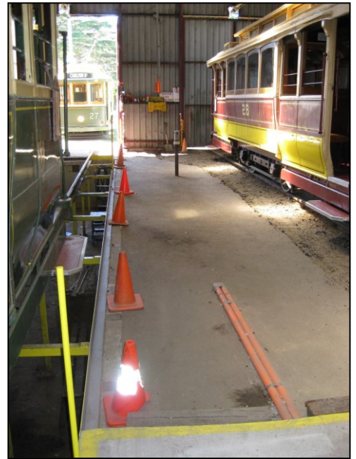
Above: Preparation for further concreting. Photo: Warren Doubleday (12/10/14)
