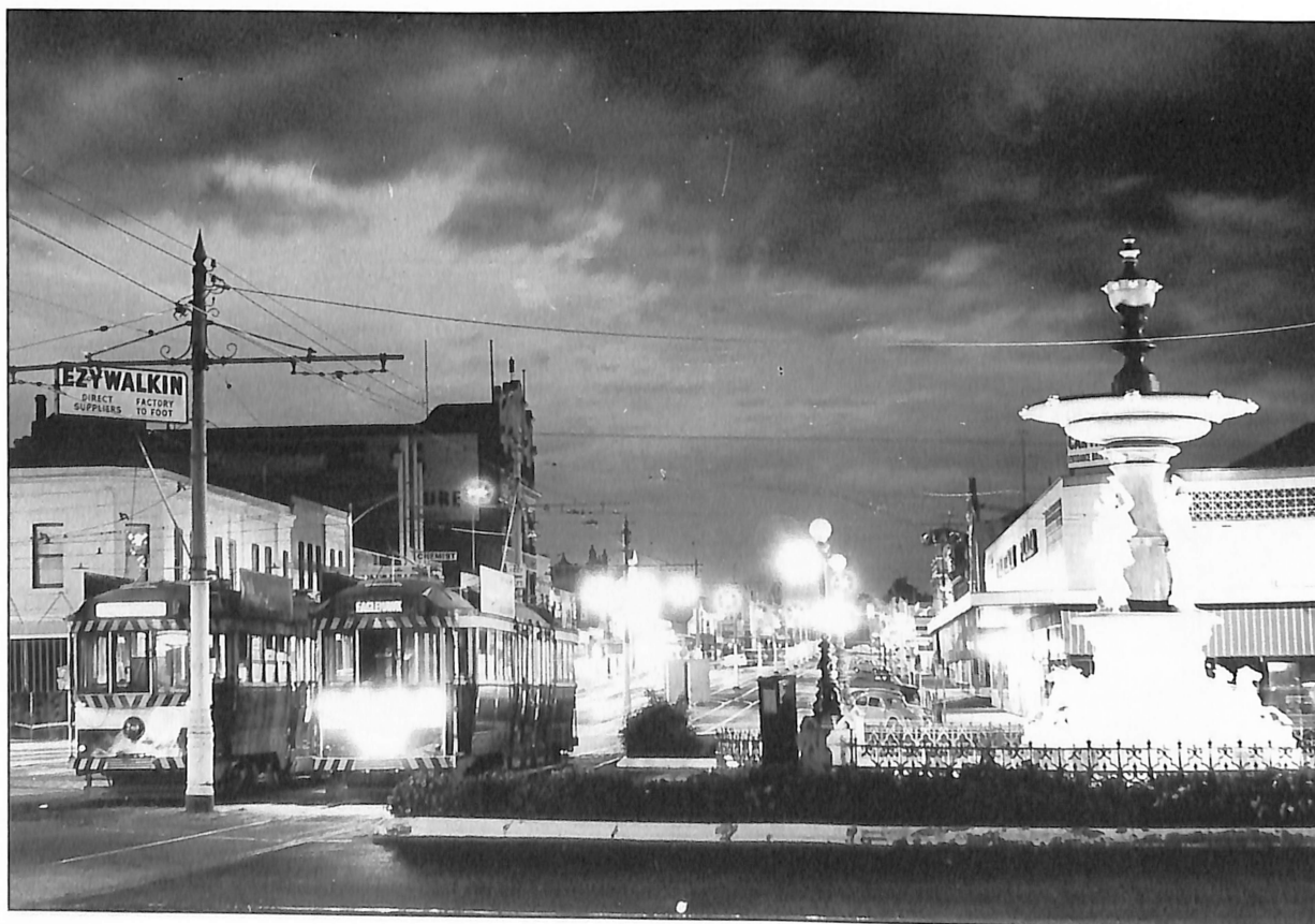
A night view of Charing Cross. Comparison of the car ends indicates the improved lighting arrangements added by the Commission to make the cars more visible after dark and thus reduce accidents. 1971.
