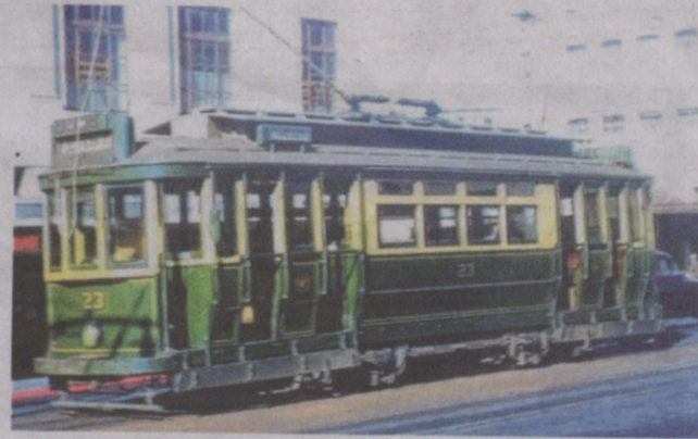
A tram in the city passes the now condemned Belchers Building on the corner of Moorabool and Ryrie streets.
