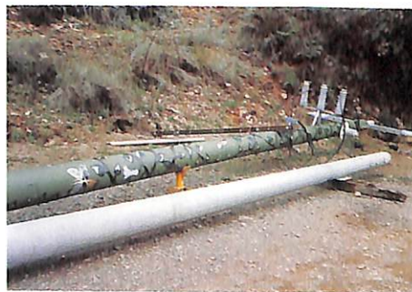
▲ The painted power pole.
