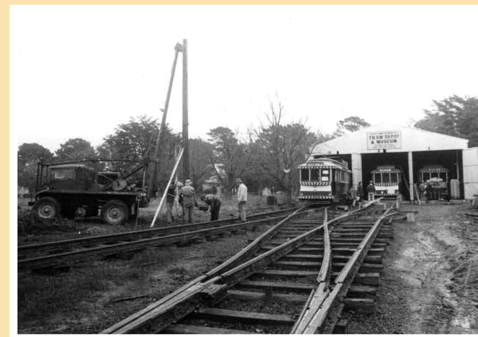
Track and electrical supply under construction. Photo: Bob Prentice, 8 April 1973
