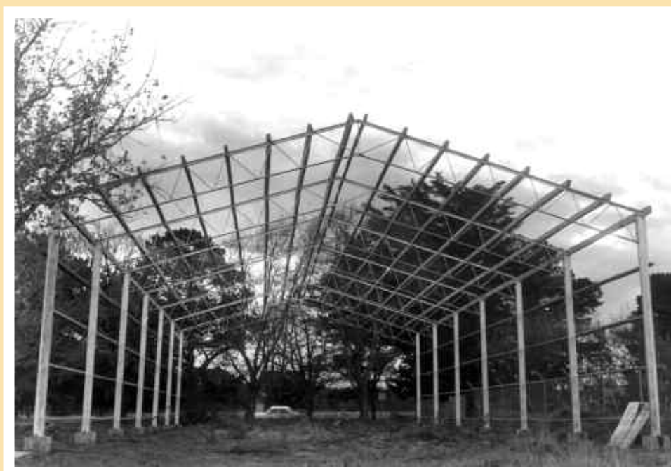
Museum's depot under construction. Photo: Ballarat Courier, July 1972
