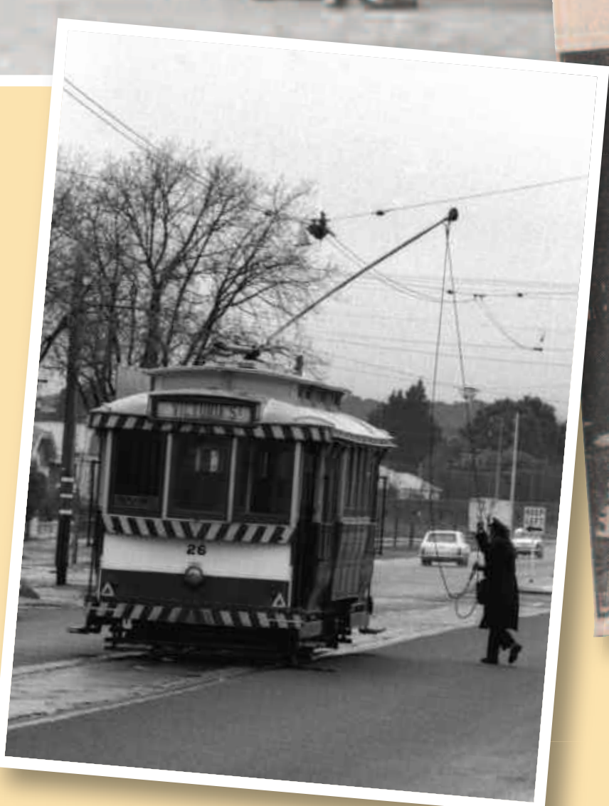
Left: Turning the pole on a tram at the terminus was a risky job on the then Western Highway from Melbourne. Photo: Peter Bruce, 1970
