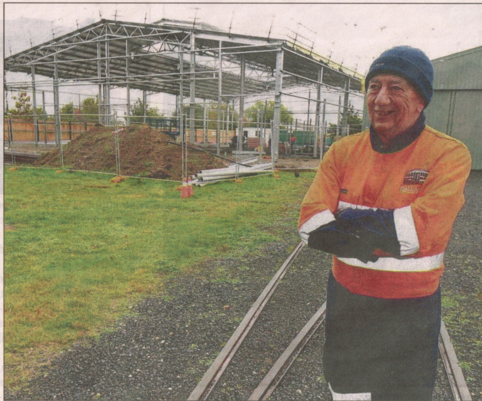
INCOMPLETE: Ballarat Tramway Museum volunteer Chris Phillips outside the site of the new museum building. Picture: Lachlan Bence
