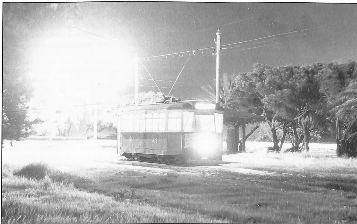
X 2 675, Point Ormond, three nights from the closure of the VR line. The full 600 volts having been restored, cars need TWO trolley poles to handle the voltage. 25.2.59.
