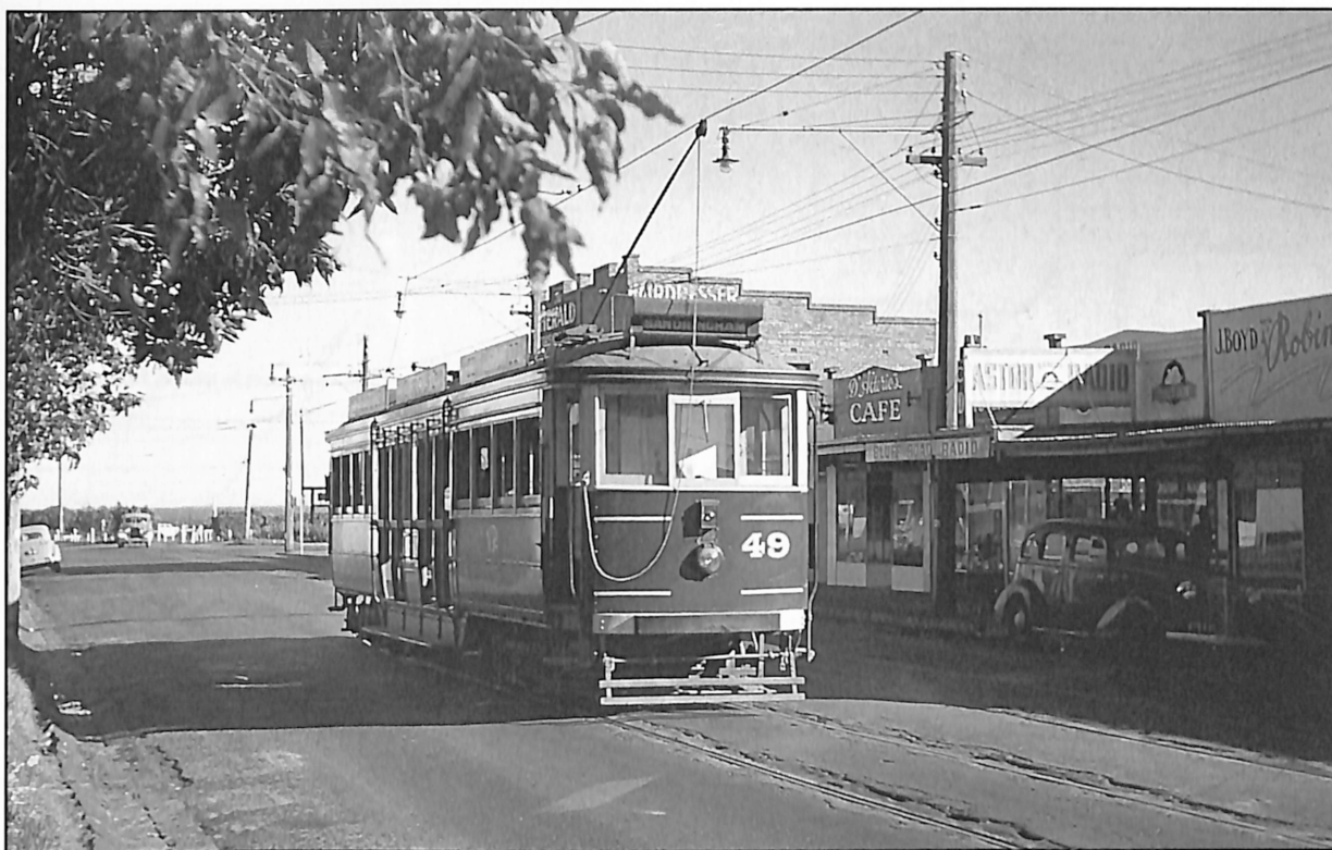
The Black Rock tramway which commenced in 1919 ran a further 2¼ miles to Beaumaris from 1926 to 1931. The single line extension wandered along unmade streets through the beachside sand dunes, serving at that time a sparsely settled area. The tea trees and dunes have ironically given way to development, becoming one of Melbourne's most exclusive suburbs. At the Black Rock terminus in Bluff Road, 49 is arriving from Sandringham. June 1956.
