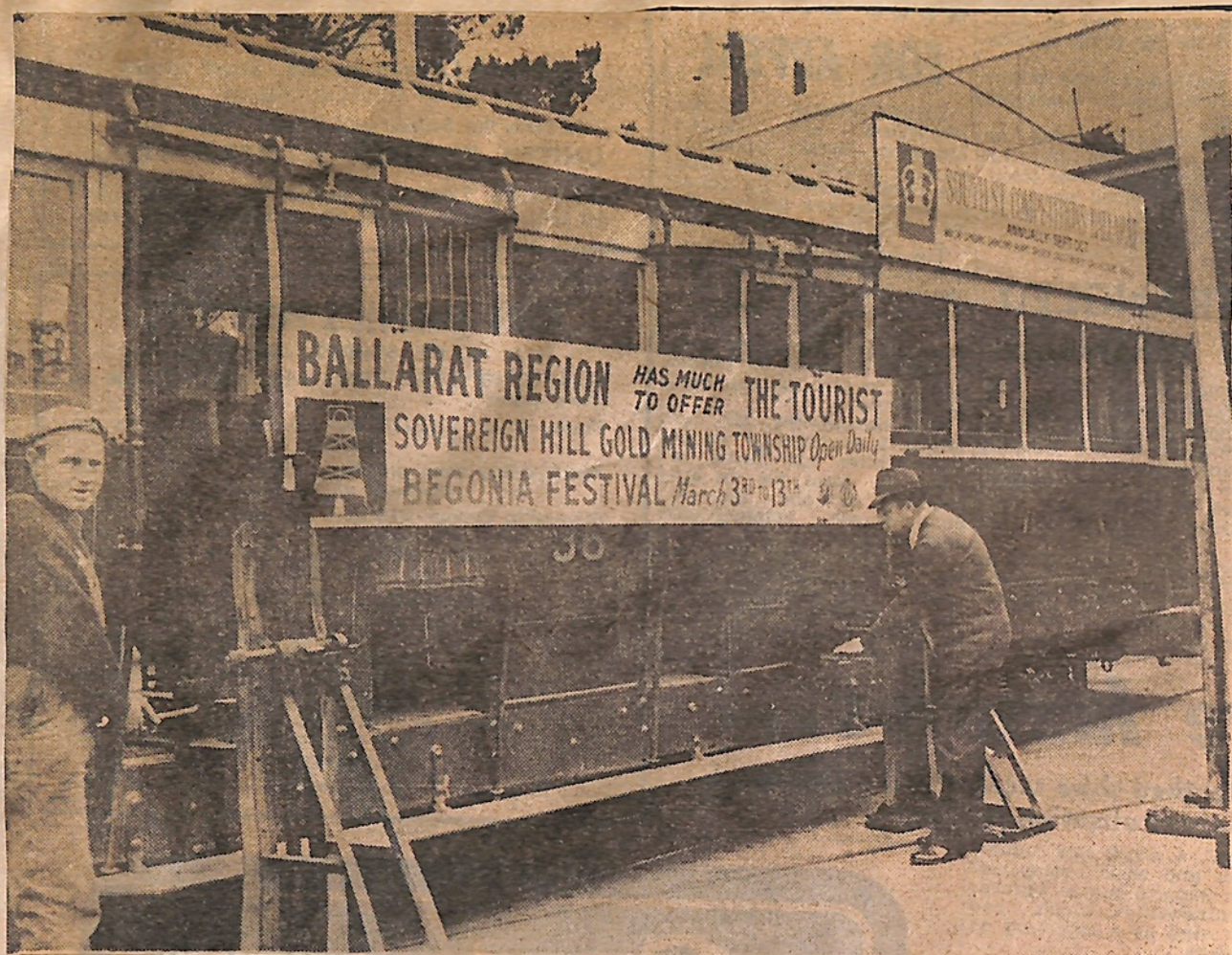
Mr Doug Wiseman, left, and Mr Bob Prentice jack up the tram to load it for transport to Melbourne. After the tram has run in Melbourne for a week, advertising the Begonia Festival Sovereign Hill and the Royal South Street Competitions, it will be retained by a Hawthorn preservation society.
