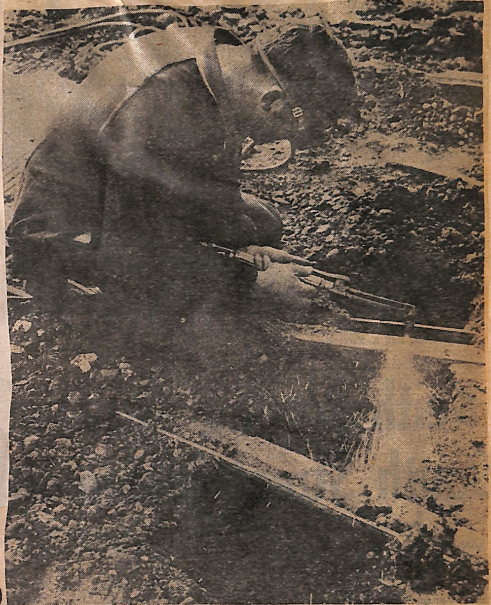
The end of the tram era was made even more apparent yesterday when welder K. Drever, of the Country Roads Board, began cutting tram lines in Sturt street.
