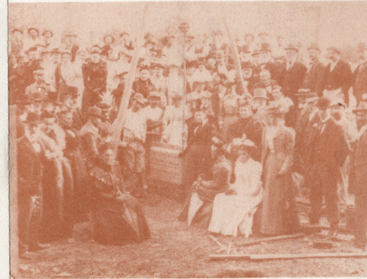
Laying the Foundation Stone of the Queen Victoria Block, 1897.
