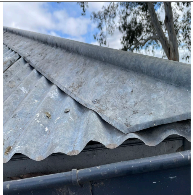
General ridge capping in acceptable condition.
