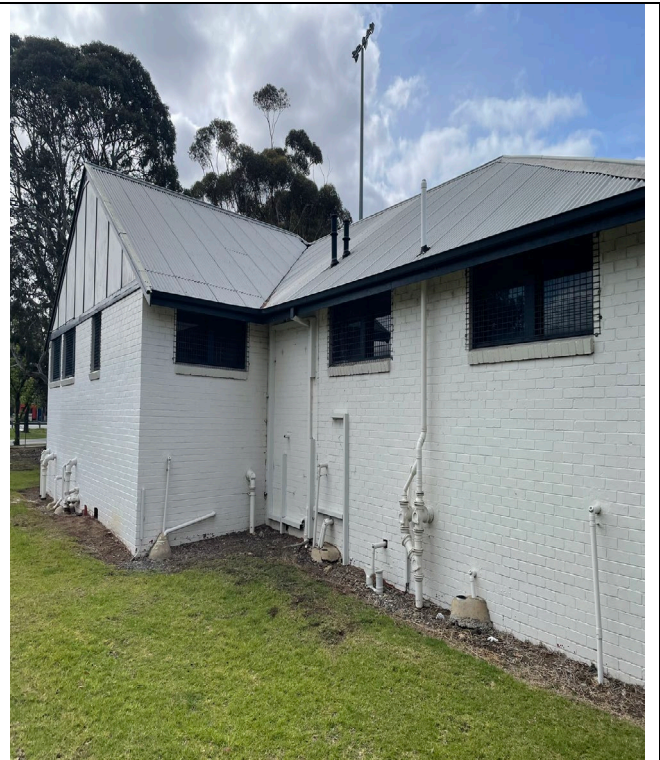
Rear elevation with articulation of masonry joints at wall interface.
