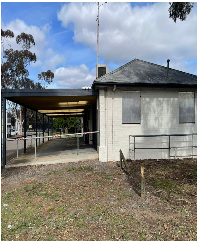
Attached Verandah to front elevation of building.
