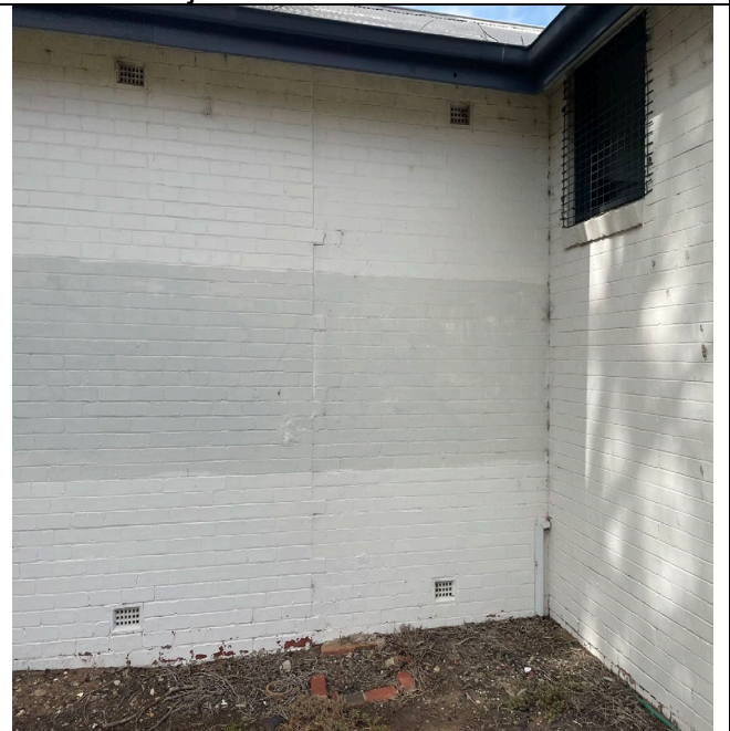
Rear elevation with articulation of masonry joints at wall interface.
