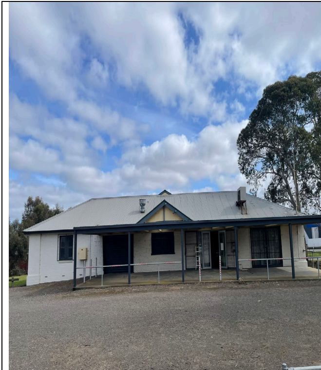
Overall structure of masonry walls with corrugated metal roof. Acceptable condition.
