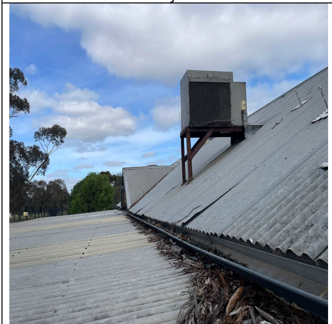
Propped valley construction. No sarking or insulation layer evident.
