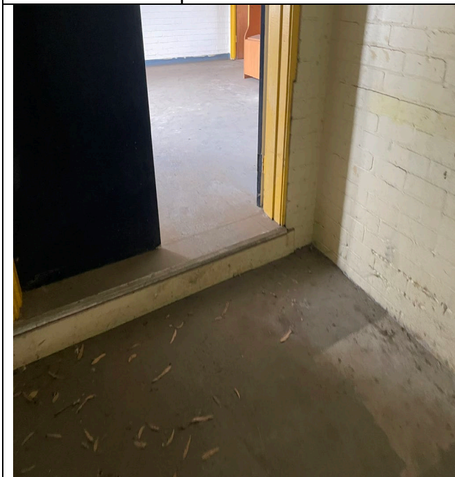
Exposed concrete slab areas to the changing rooms in acceptable condition.
