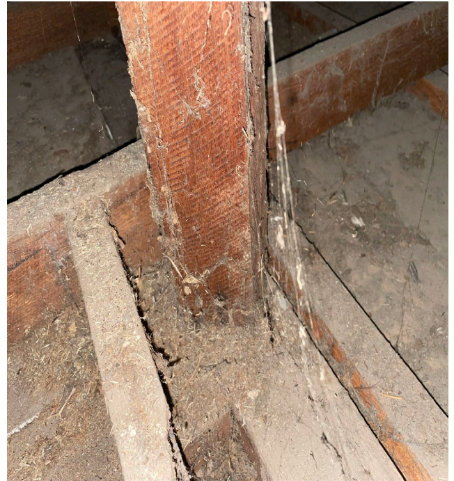
Props onto masonry loadbearing walls.
