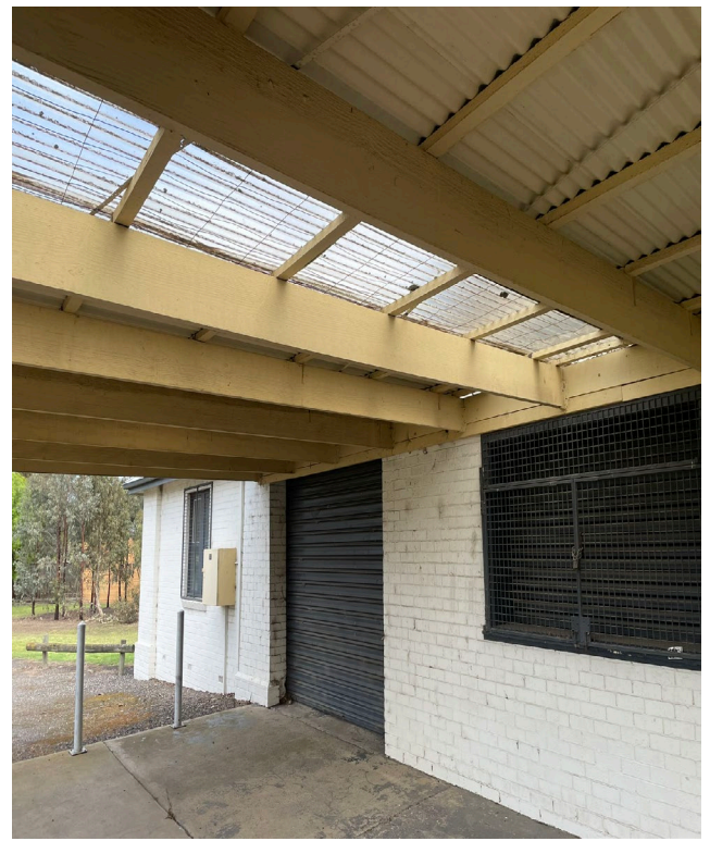
Members connected using proprietary joist hangars with battens and sheeting over.
