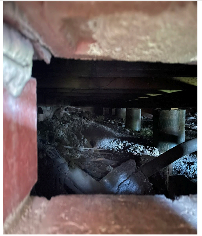
Concrete piers supporting suspended concrete floor areas
