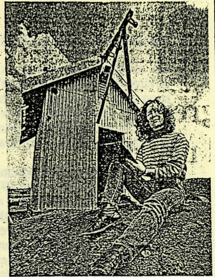
DUNNY ON THE HILL . . . The old electricity sub-station behind student Anne Kershaw was dubbed 'dunny on the hill' by the locals when it was built early this century to generate the main power for the pipeworks. PICTURE: LISA BIGELOW
