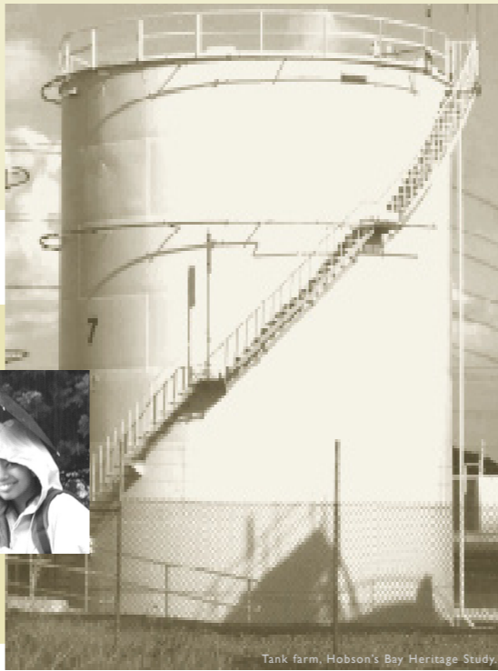
Tank farm, Hobson's Bay Heritage Study.
