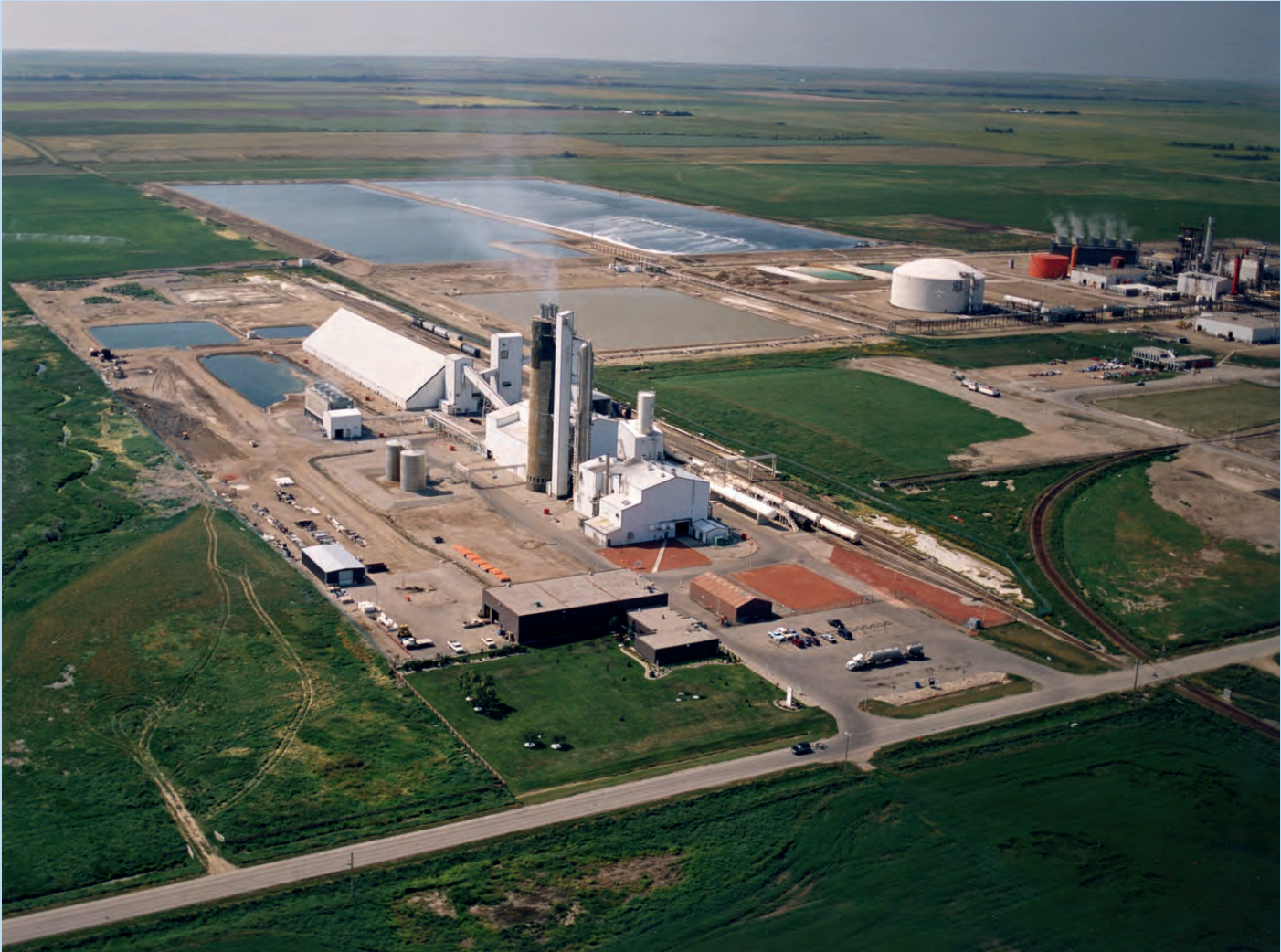
Orica's Carseland ammonium nitrate manufacturing centre in Canada.
