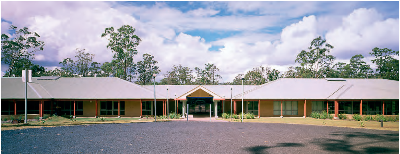
Orica's Technology Centre in Kurri Kurri, New South Wales.
