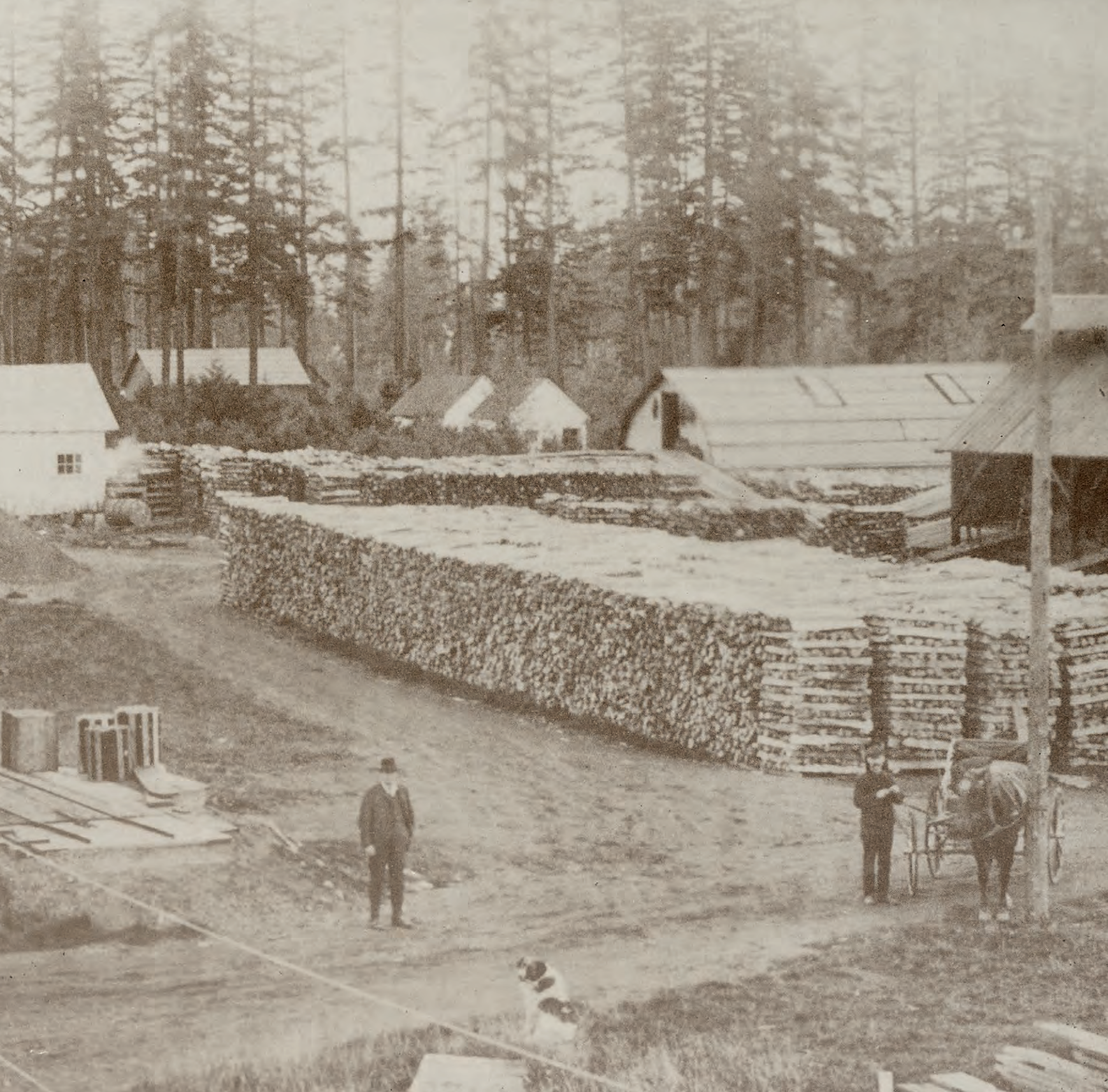
The wood yard and kilns for the production of charcoal used in the manufacture of black powder at Deer Park, Australia.
