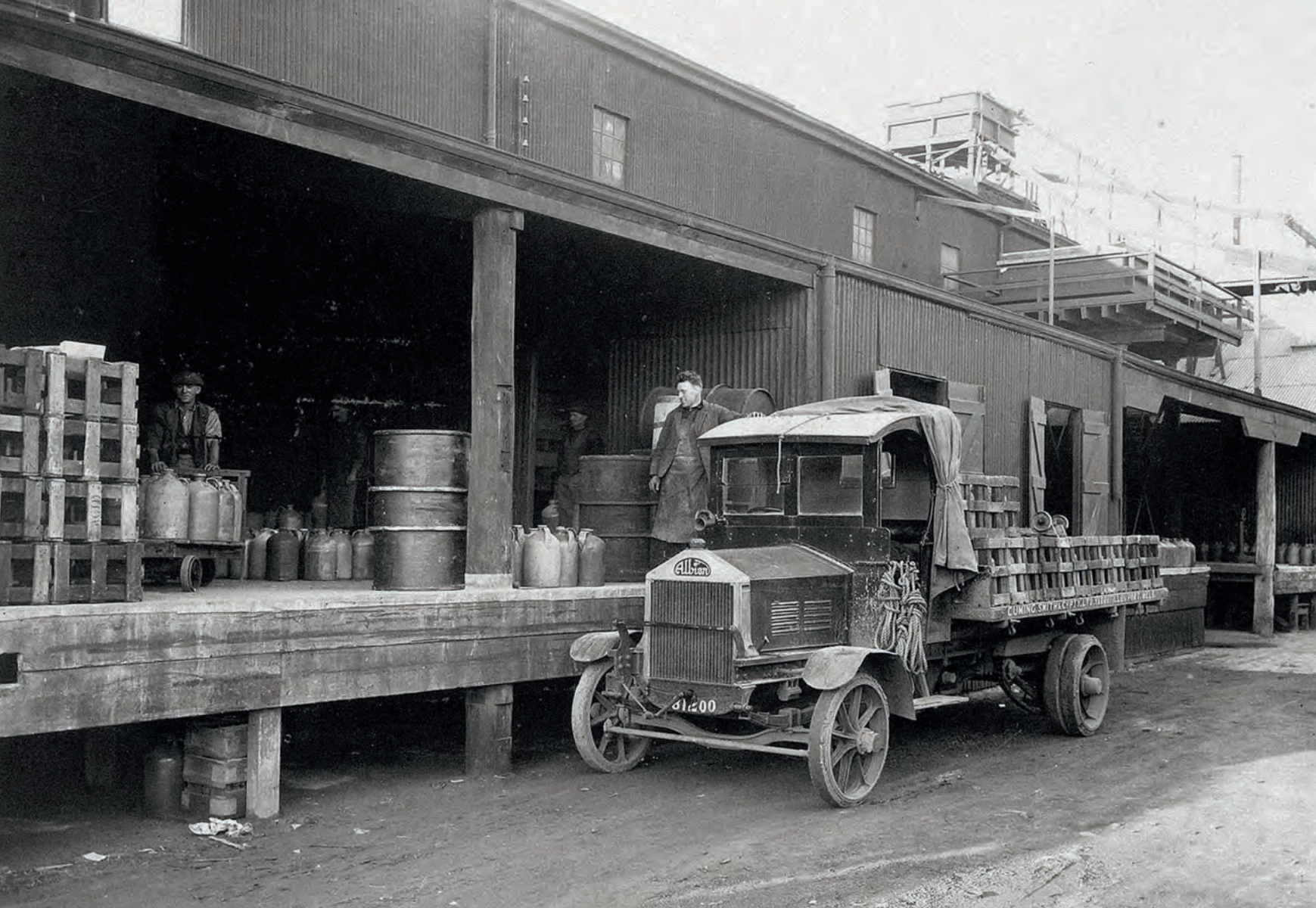
Loading the truck for deliveries at the Yarraville site.
