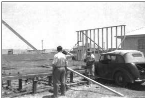
House construction Alfrieda Street © K Haumann
