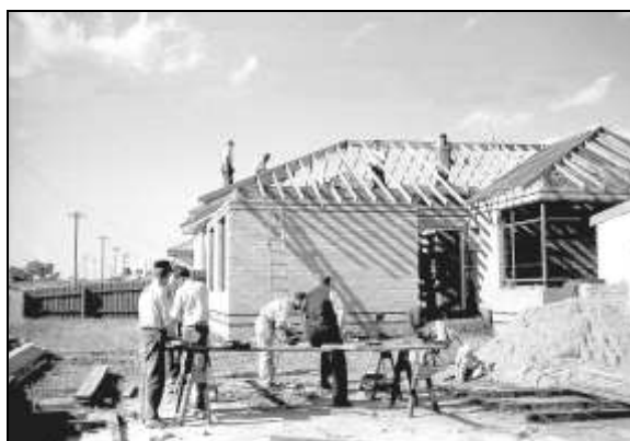
Putting on the rafters © Kon Haumann
