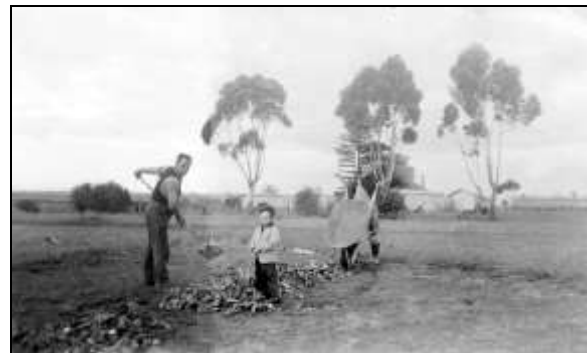
Wilhelm Stein repairing potholes © Mary Smith
