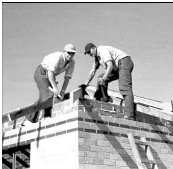
Putting on the rafters © Kon Haumann
