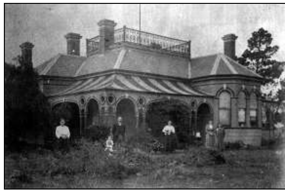
Padley home in Winifred Street, built circa 1887
