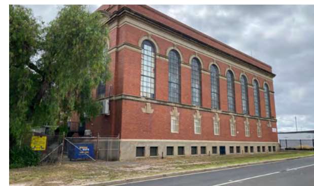
The former substation provides a significant opportunity to define character and needs to be integrated sensitively.
