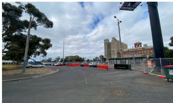
The station surrounds are dominated by car parking, with little consideration for how pedestrians navigate the space.
