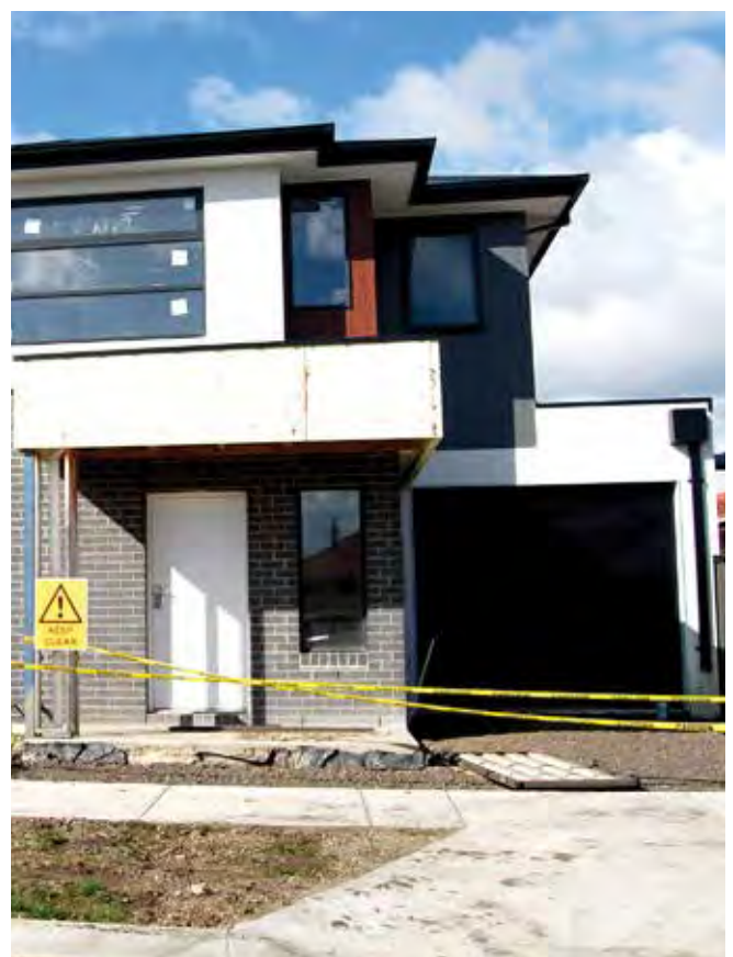
NEW HOUSING UNDER CONSTRUCTION IN DEER PARK
