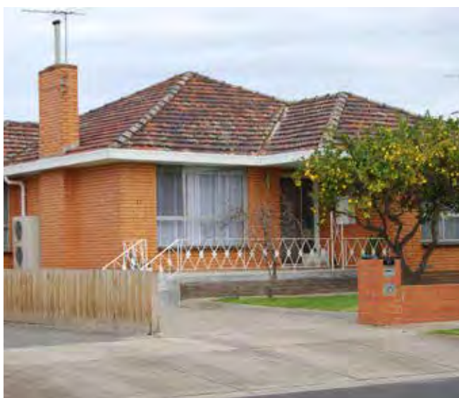
BRICK DWELLING, WESTWOOD WAY, ALBION
