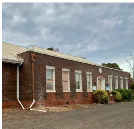
Heritage Building on Site
