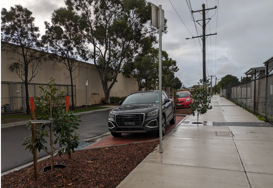
Better Streets for People Project upgrade complete at George Street, Sunshine including increased footpath width, tree planting for shade trees and passive irrigation.
