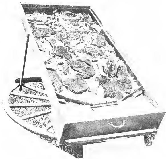
Fig. 14.—SOLAR WAX EXTRACTOR.
