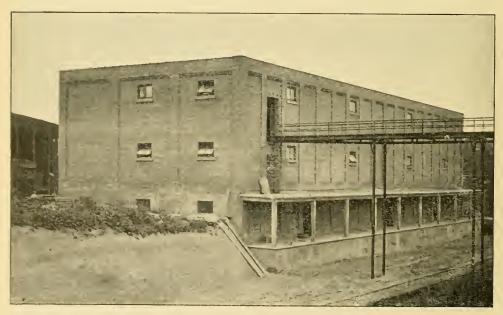
The A. I. Root Company's Fire-proof Warehouse, 148x48, three stories, with loading-platform and steel bridge connecting old Warehouse on the south.
