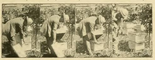
METHOD OF INSERTING THE ESCAPE-BOARD.
