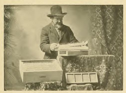
THE YODER PLAN OF FASTENING FULL SHEETS AT THE TOP AND TWO-THIRDS THE WAY DOWN THE SIDES.
