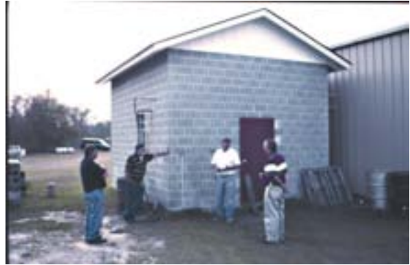
This concrete block building has been built to house a tank to store high fructose corn syrup. The operation utilises between 23-24 thousand lbs of syrup per year. Stored in warm conditions to prevent crystallisation. Reg Wilbank's honey house, Georgia.
