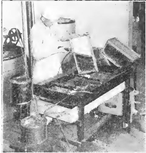
Uncapping combs with a steam-heated uncapping-knife.
