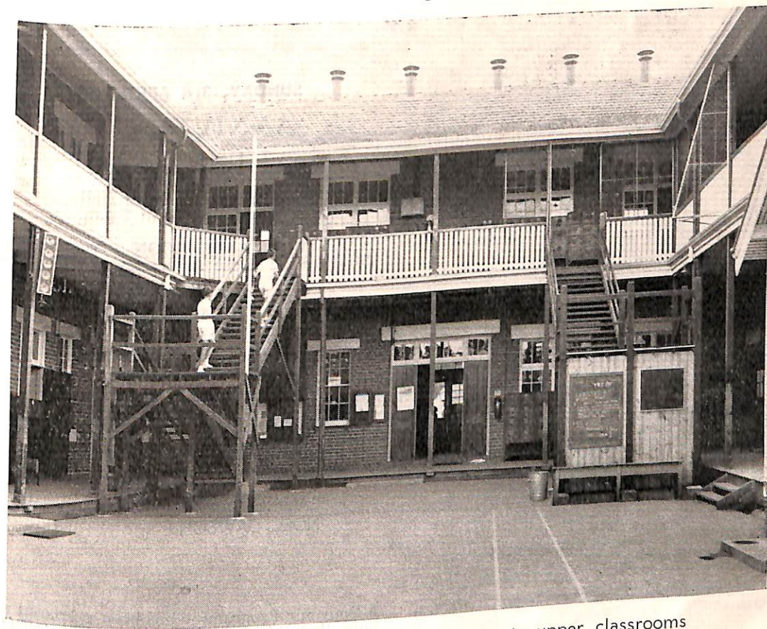
A view of the Quadrangle, showing new stairways to upper classrooms
