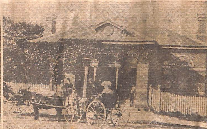
YOU CAN STILL recognise the Dandenong Post Office of today from this old photo, taken about 50 or 60 years ago. The main P.O. building, despite its additions, is basically the same today —except in those days it did have a clock!
