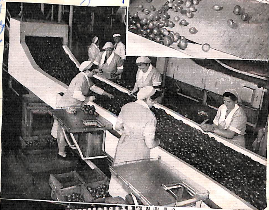
Top:—An automatic tipper sends tomatoes tumbling out of their crates at the start of the canning process.
