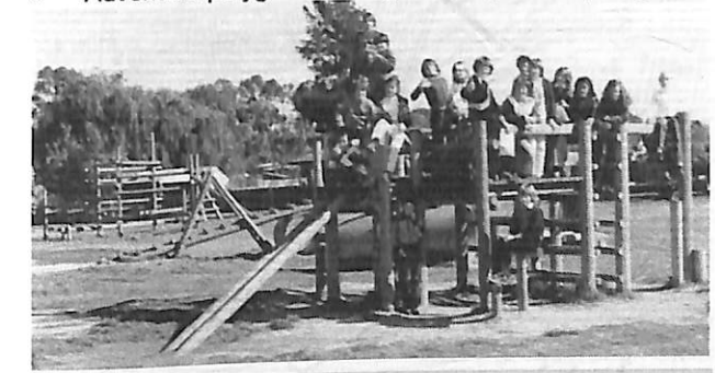
Adventure Playground: Following a co-operative arrangement with the then City of Springvale a fine adventure playground was constructed in 1975, near the northern boundary adjacent to where a supermarket car park was later established. The play equipment, of treated pine, was financed on a dollar for dollar basis with the Springvale council. A pine bark base was added in 1981.
