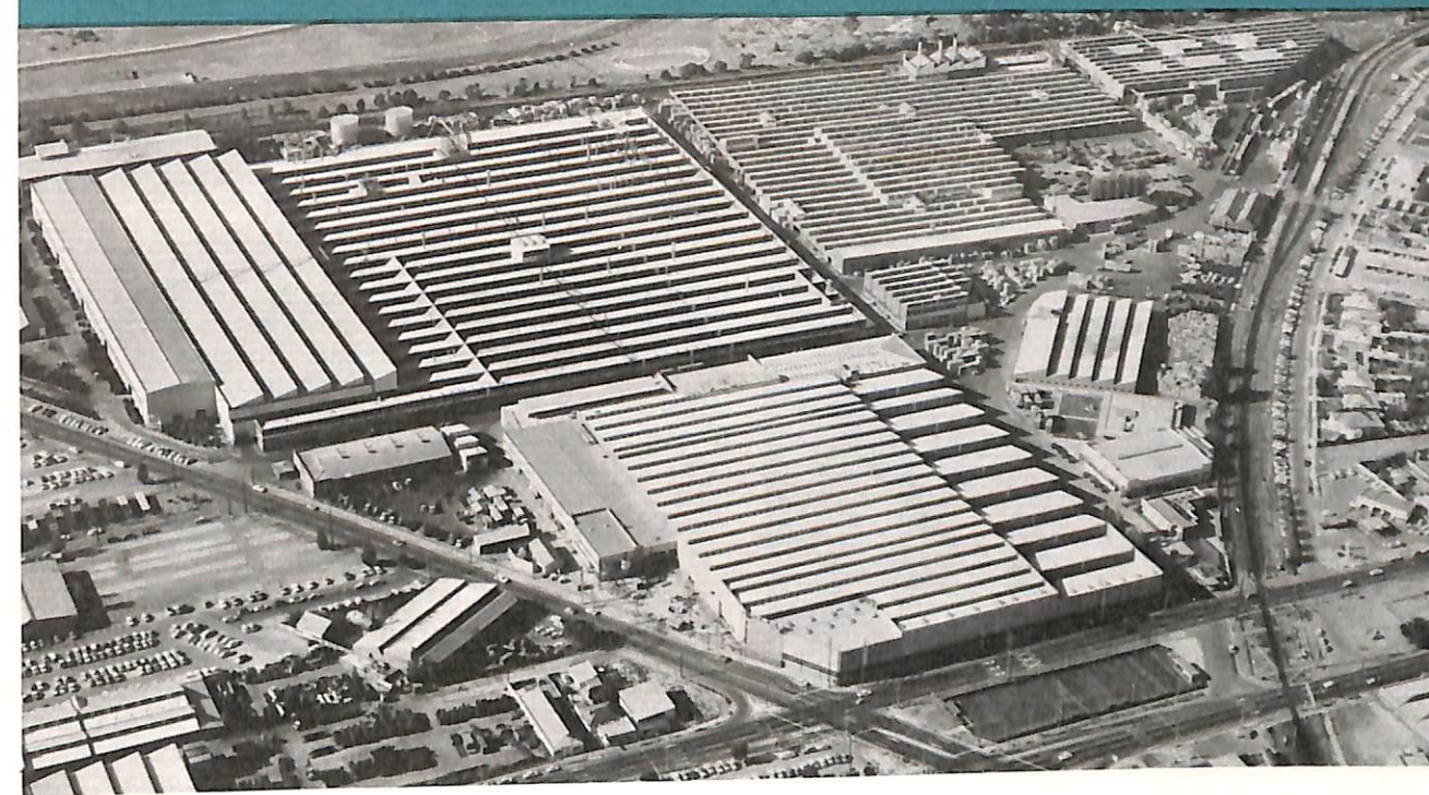
Woodville, South Australia, where tools, welding fixtures and dies for metal stamping and body building are produced. Here also GMH produce body components and plate Holden bumpers and other parts.
