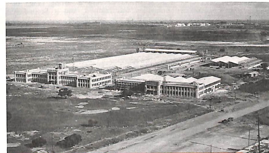
Under direction from the Fishermen's Bend Plant, shown here under construction, production for 1936-37 swept up to 28,000 units, representing 40 per cent. of the market.
