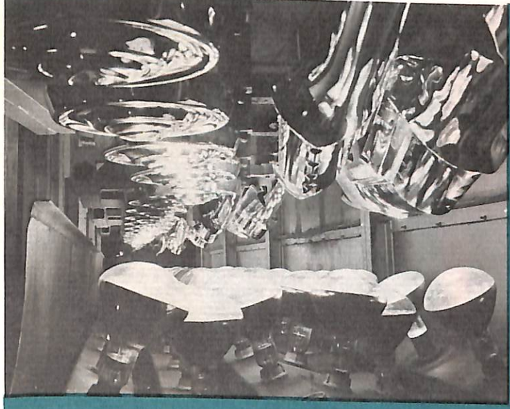
Electro-plating wheel hubs and body hardware at the Woodville Plant.
