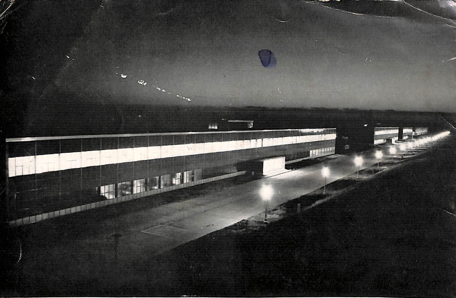
ABOVE:— Night photo of facades of Dandenong Plants of GMH.
