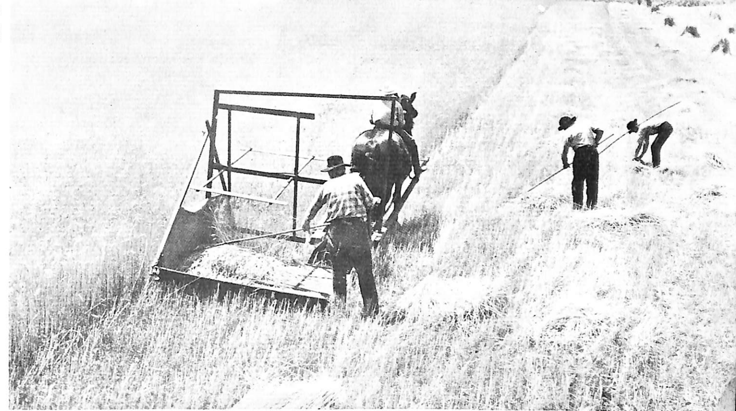
With the invention of the world's first practical reaper by Cyrus Hall McCormick in 1831 farm mechanization took a step forward far greater than ever before. This machine would cut as much grain in one day as four or five men with cradles—as much as 12 to 16 men with hand sickles. Within a decade the time required to harvest an acre of wheat was reduced from about 37 hours to an estimated 11½ hours, with a big decrease in the use of physical labour.
