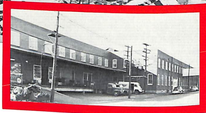
Close-up of main administrative block
