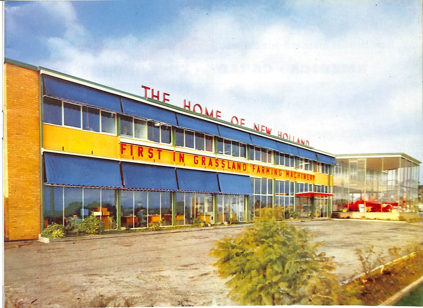
Administrative block at the Dandenong (Victoria) factory and Head Office of New Holland (Australasia) Pty. Ltd., Division of Sperry Rand Corporation, U.S.A.
