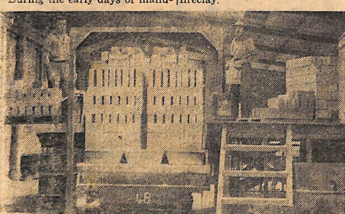
BRICKS at the Ordish works are stacked on a tunnel car before entering the dryer and tunnel kiln. Spaces between bricks allow free flow of hot air. The frame serves as a load limit.
