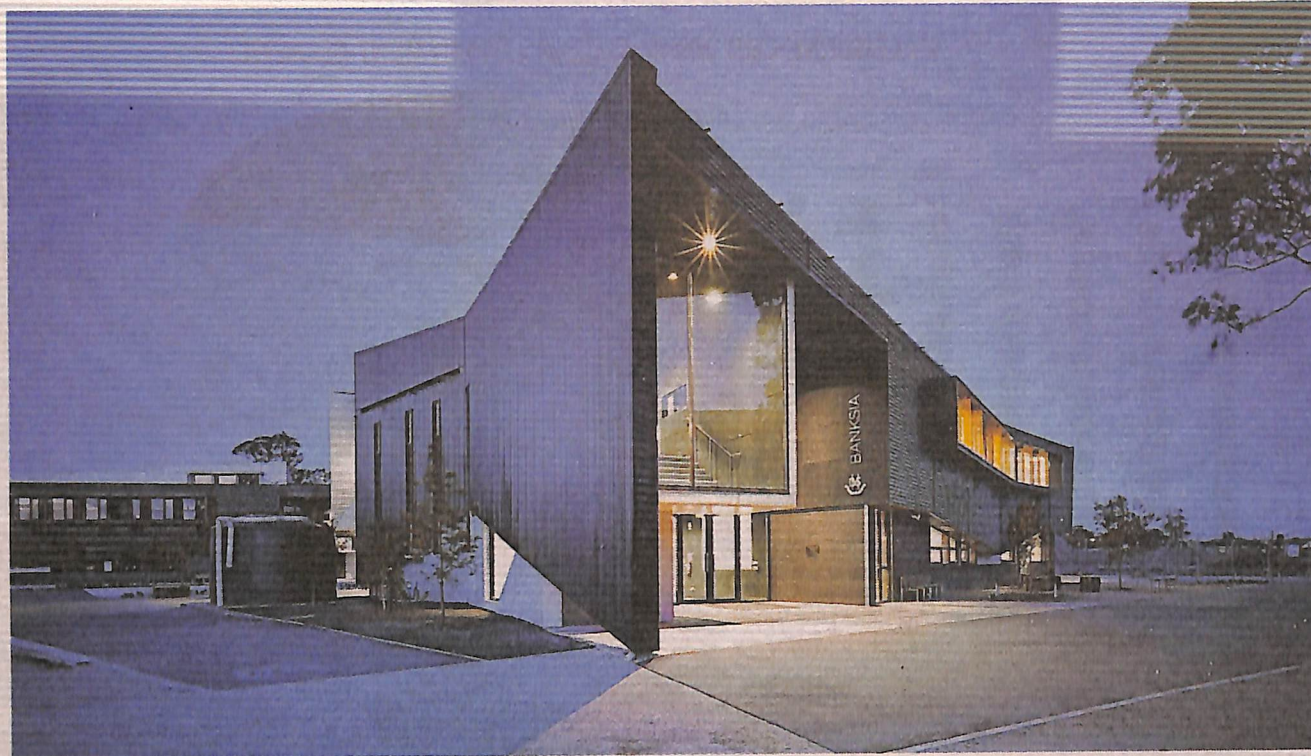
The southern facades are finished in black steel, while the northern ones are clad in white.
