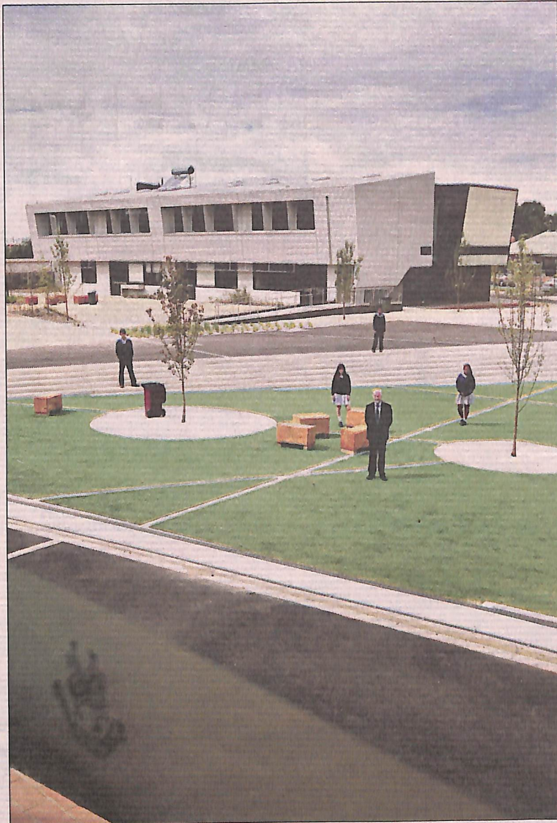
The latest stage of the Dandenong High redevelopment is complete. Pictured outside the new building are Principal Martin Culkin with year 10 students Romal, Mani, Albiona and Prarthana. Picture: VALERIU CAMPAN N350S102
