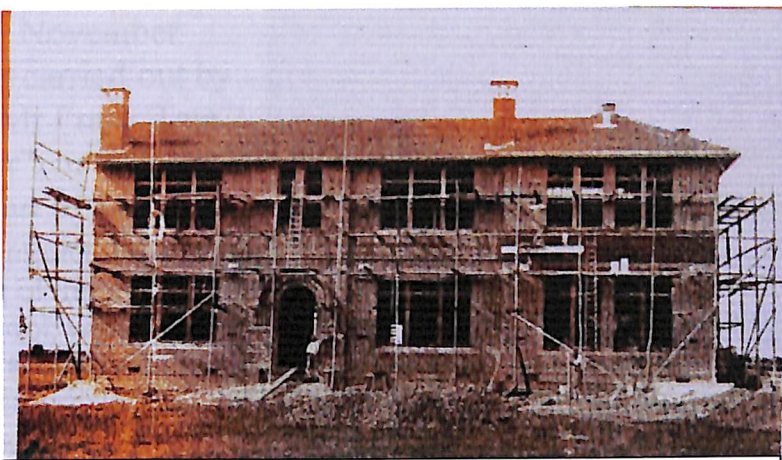
Front classrooms under construction, minus the west (left) wing, added a short while later
