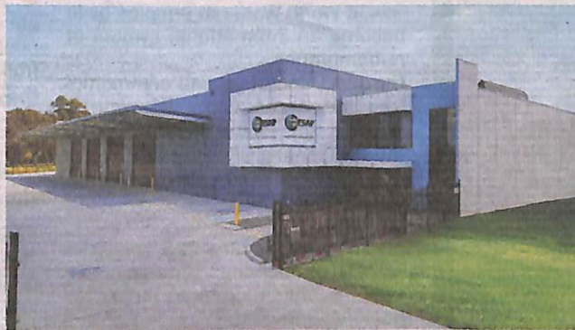
ESAP's new Keysborough facility.
