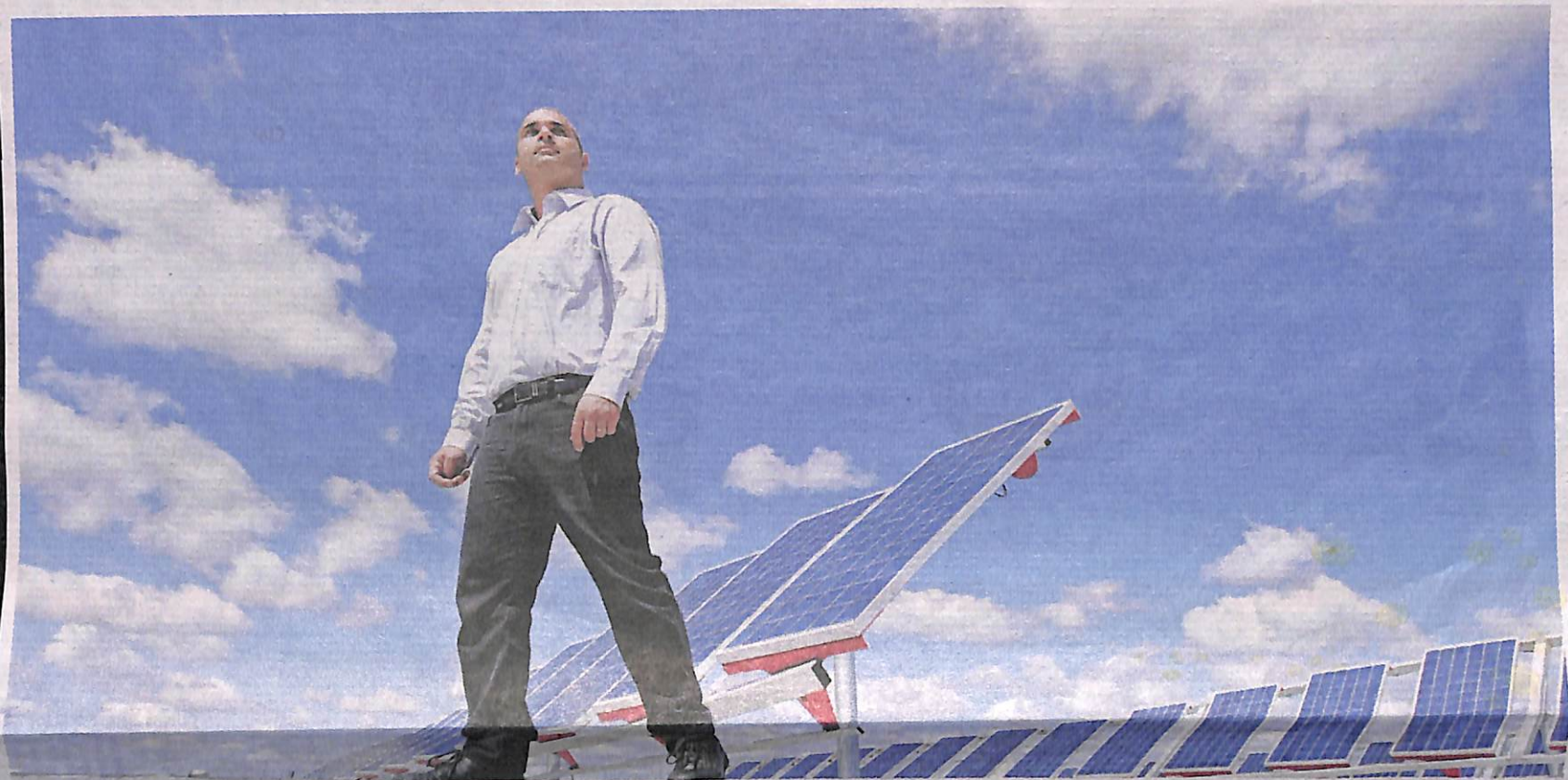
Project manager Jacques Esper surveys the solar set-up on the roof of Hilton Manufacturing.
