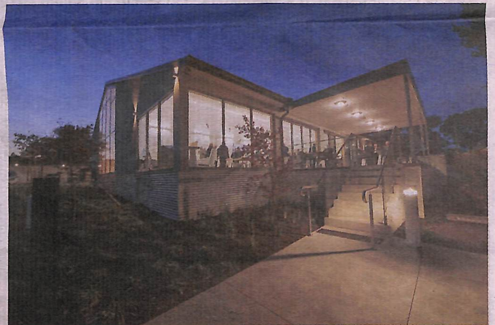
The home casts a welcoming glow at night.
