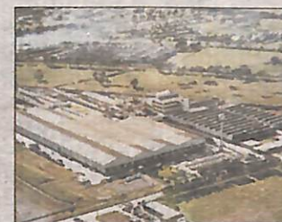
From the top: A shot of the Pilkington site.
