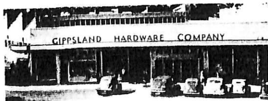
GIPPSLAND HARDWARE COMPANY. This modern store has just been completed and was opened for business last week in Lincolne Street — Dandenong's main thoroughfare.
