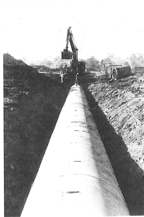
Pipeline Construction Works.
