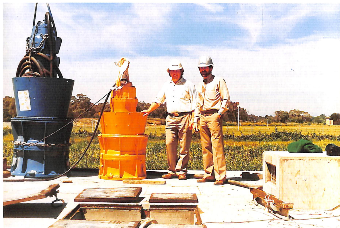
Submersible pumps for Kananook Creek Pumping Station.
