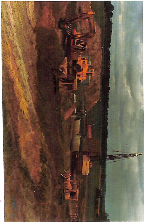
Construction of concrete lined channel utilising concrete paving machine on Dandenong South Drain.
