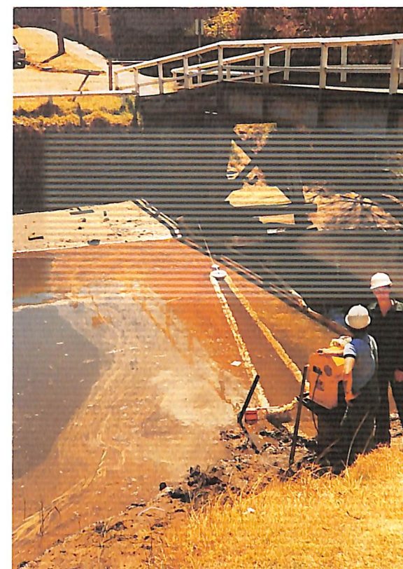
Removing Pollution spill in Kananook Creek using oil mop.
