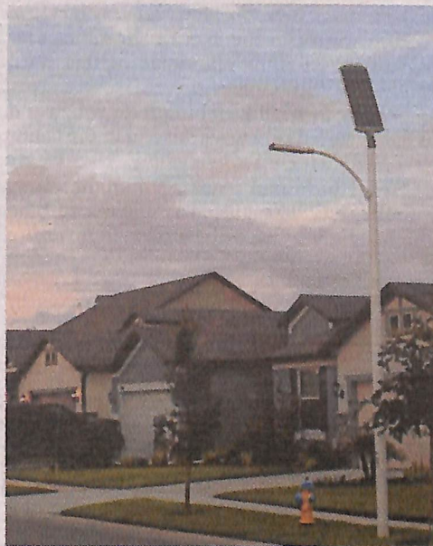
One of the smart solar lights, which can store power for days and be controlled remotely anywhere in the world.
